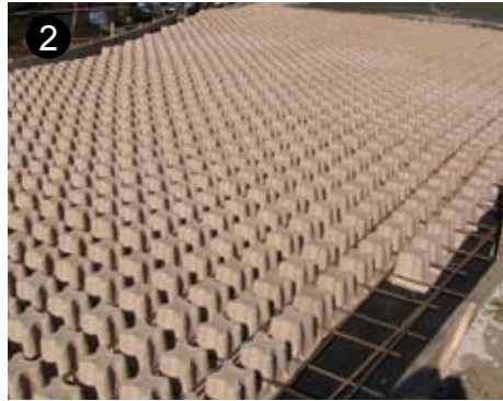
Grasscrete Molded Pulp Former Installation
