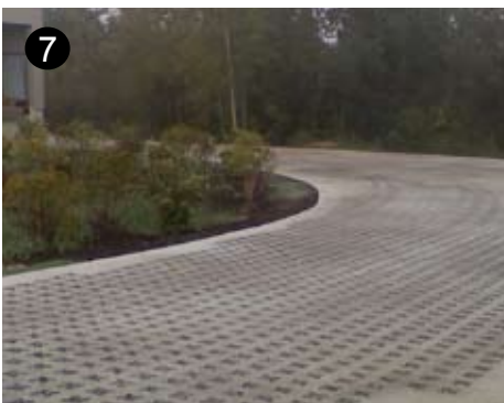
Installed Grasscrete Stone Filled Void System
