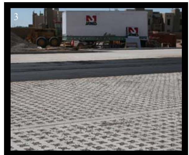
Photo 3: After concrete has been poured, broom finished and set, voids are filled with stone
