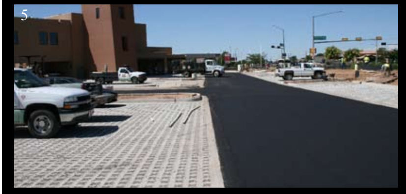
Photo 3: After concrete has been poured, broom finished and set, voids are filled with stone
